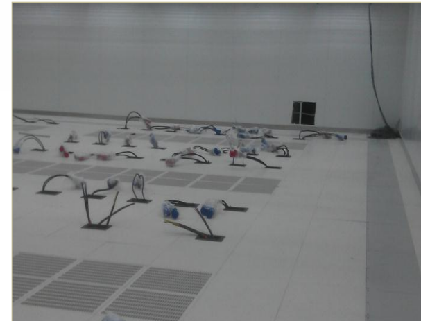
○ Completion of seismic Access double floor
