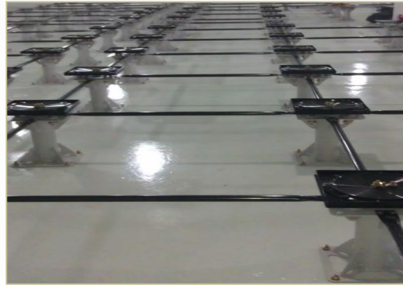
○ Supports & Links – Secondary reinforcement of seismic support
