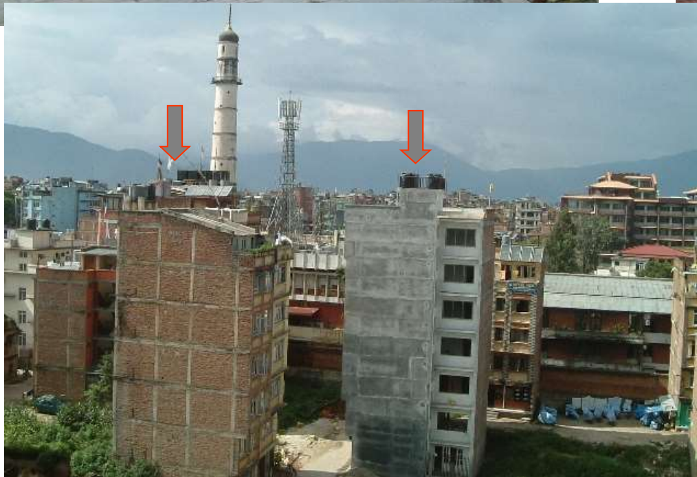
Slender buildings/houses (Improper design??)
